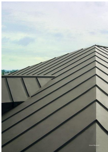
"Felsdak" in pvc-dakbedekking
